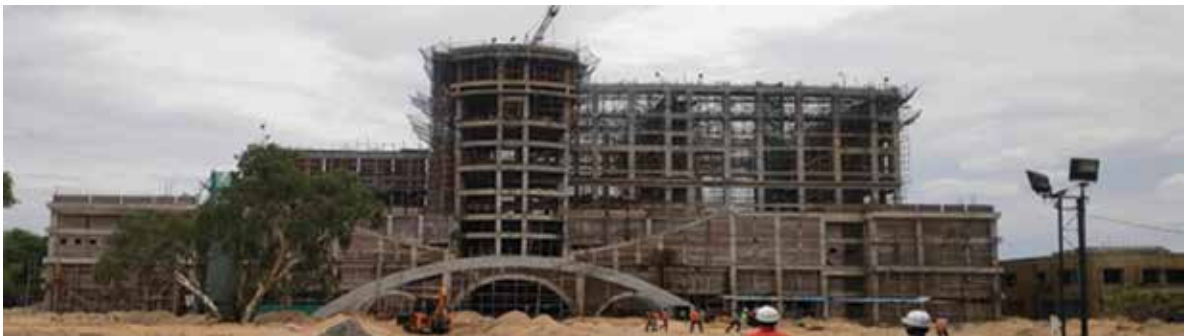
Orbital Module Preparation Facility [OMPF]
