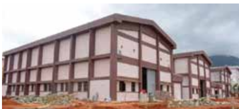
Semi Cryo Fabrication Facility
