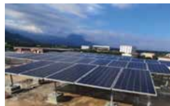
500 kWp capacity Solar Power Plants in roof top of various facilities (Under Phase-III)
