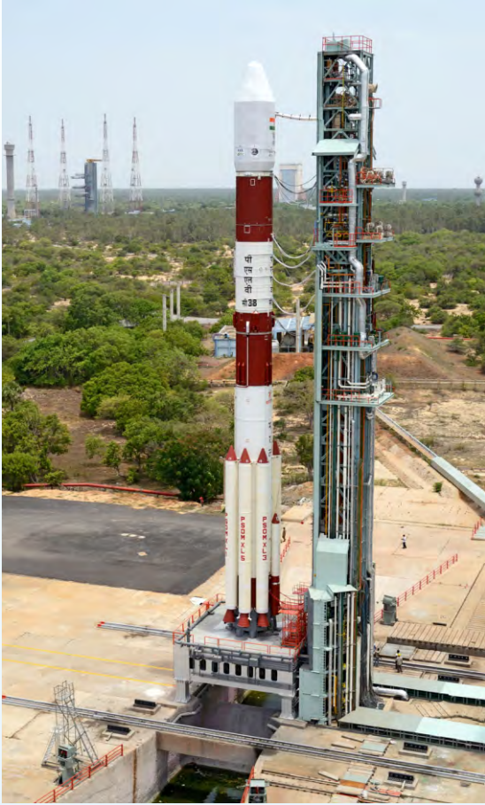
PSLV-C38 at the First Launch Pad
