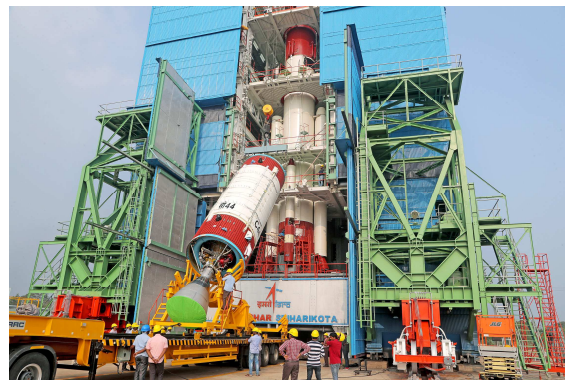
A view of PSLV-C44 second stage at MST during vehicle integration
