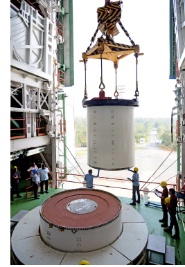
Joining of two segments of PSLV-C44 core stage in progress
