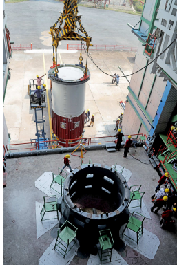
Hoisting of nozzle end segment of PSLV-C44 core stage
