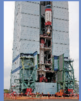
Hoisting of PSLV-C21 second stage
