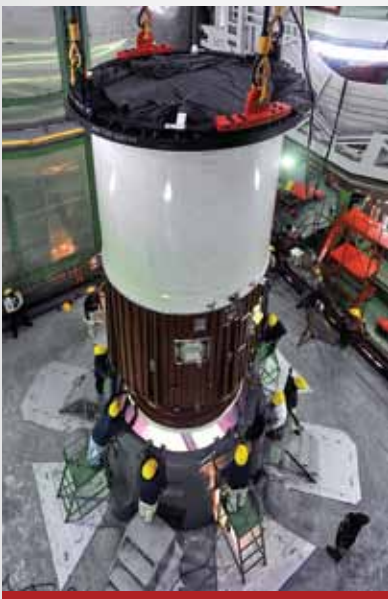
Nozzle End Segment of PSLV-C22 first stage being positioned over the Launch Pedestal
