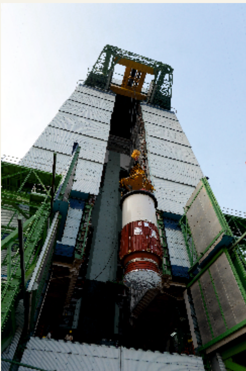
Nozzle End Segment of PSLV-C26 being hoisted for assembly
