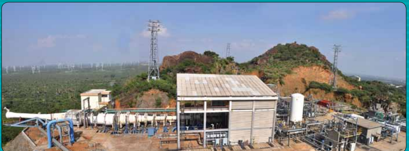
A panoramic view of Cryogenic Upper Stage HAT Facility
