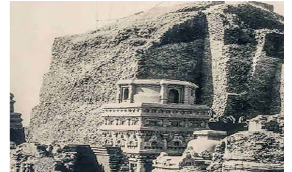
Excavation in progress 1920-1925
