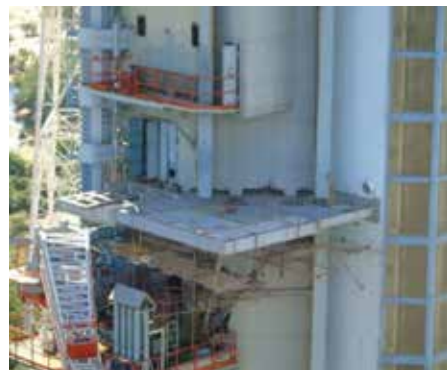
Crew Access Arm Erection at SLP-UT
