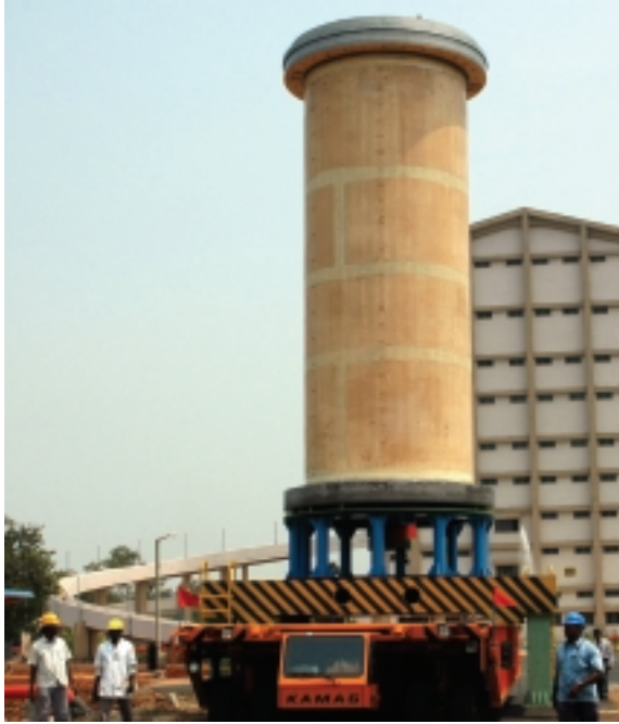
Middle segment being transported to Curing Facility
