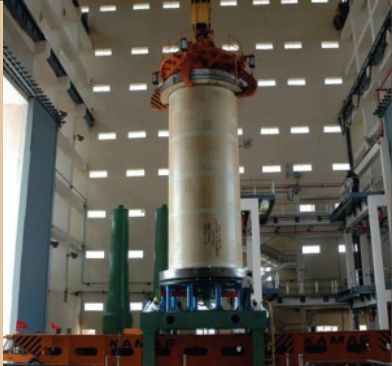
Middle segment being loaded on to the transporter
