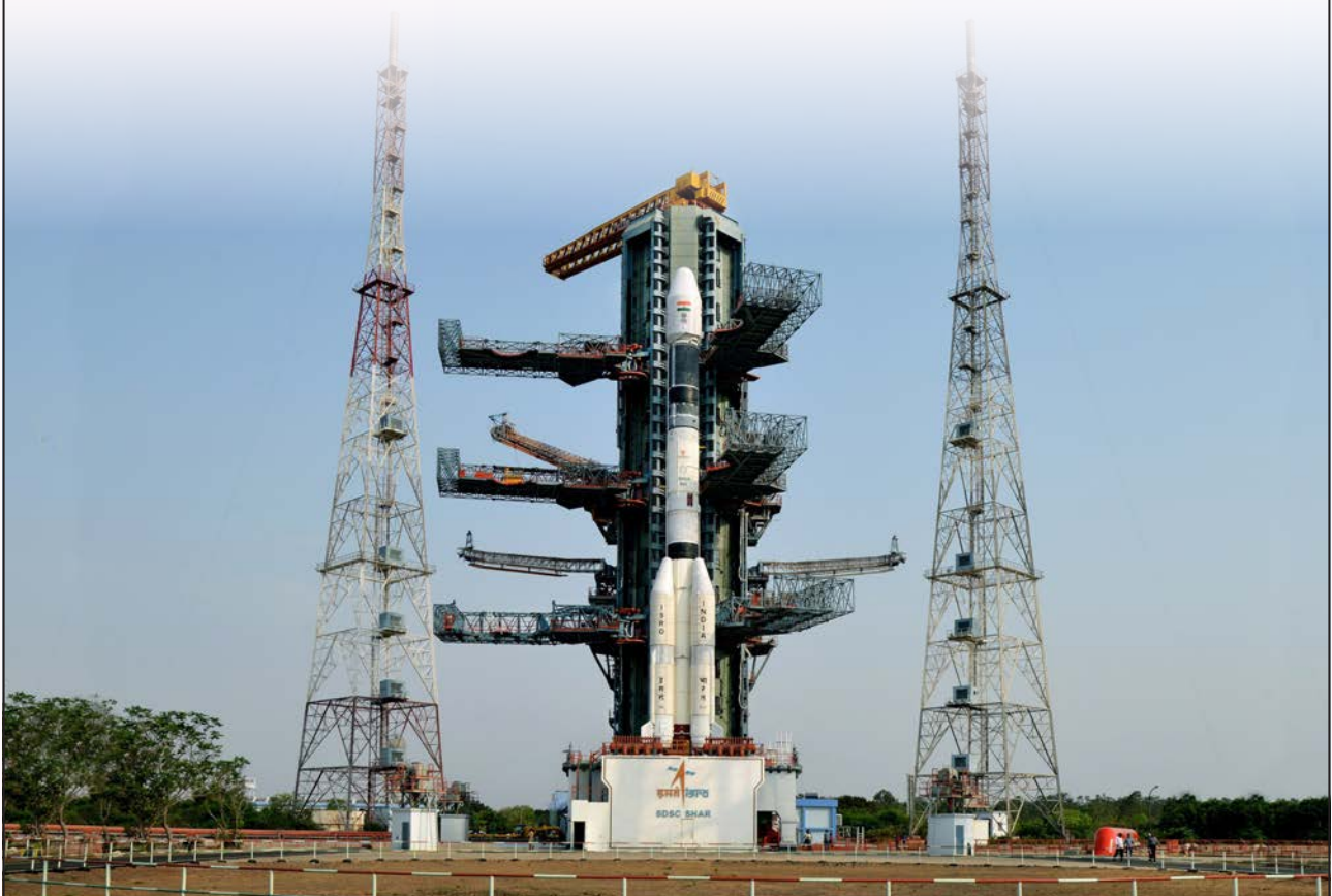
The Fully Integrated GSLV-F09 Carrying GSAT-9 at the Second Launch Pad
