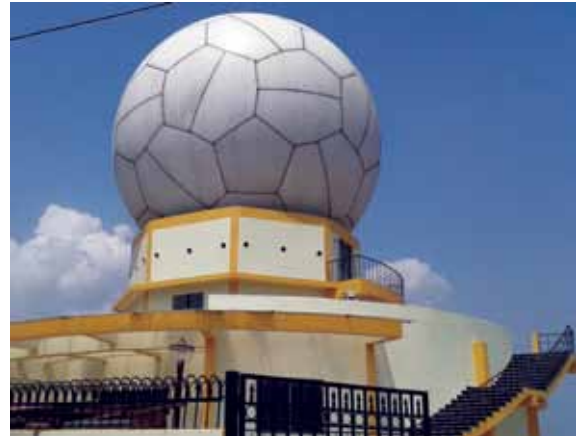
The DWR System at Cherrapunjee
