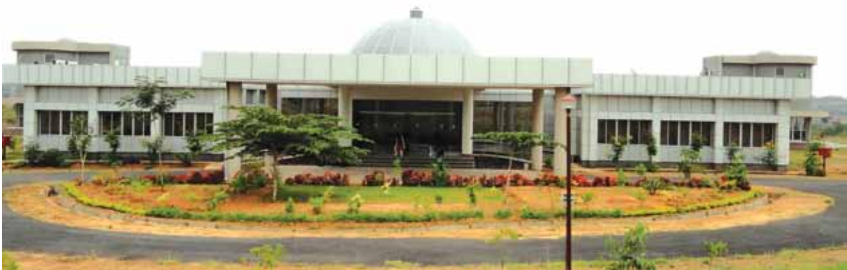
ISRO Navigation Centre (NIC) at Byalalu, the Nerve Centre of IRNSS Ground Segment
