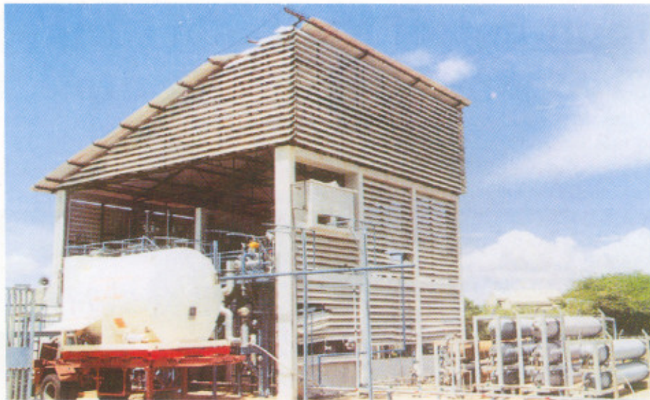
Subscale cryogenic engine test stand at Mahendragiri.
