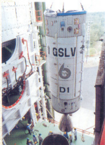
Second Stage being stacked on the first stage.
