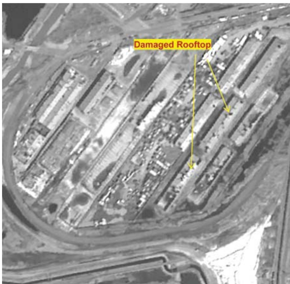
Cartosat-1 data of 16.10.2014 showing HPCL Plant with rooftops flown-off during the cyclone
