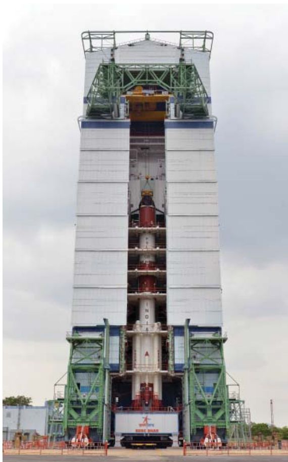
PSLV-C26 inside Mobile Service Tower prior to Satellite Integration
