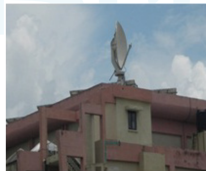
Plate.2 X-band surveillance radar
