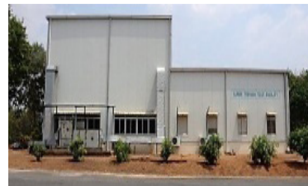
Lunar Terrain TeSt Facility
