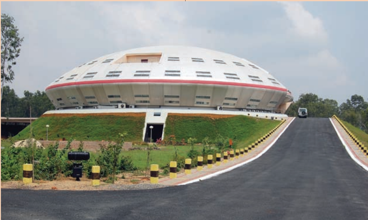
Outside view of the new Control Centre
