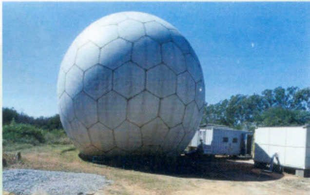
DWR installation showing the radome and other equipment located in the containers
