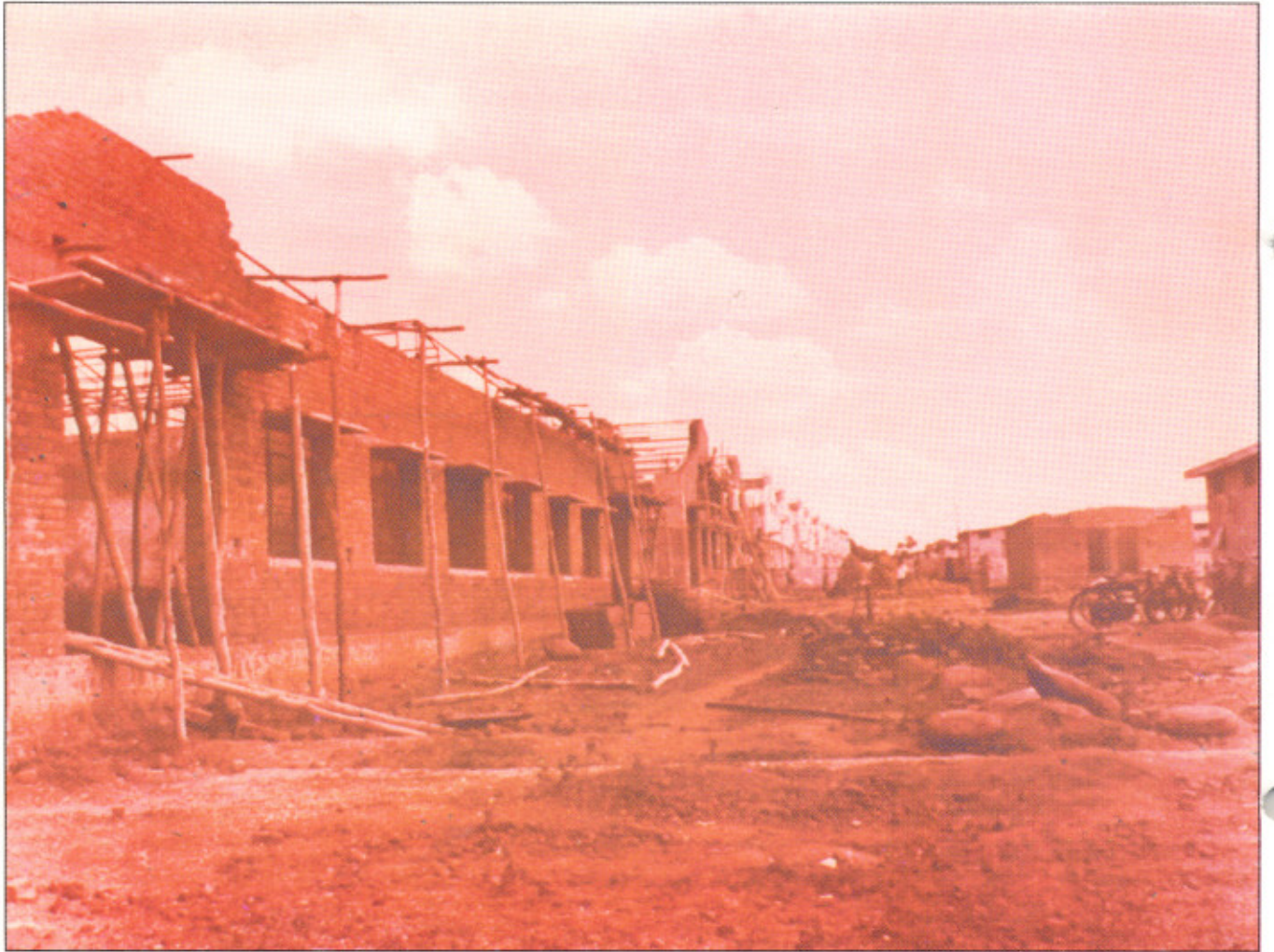
Beginning of all - industrial sheds under construction for the Aryabhata Project
