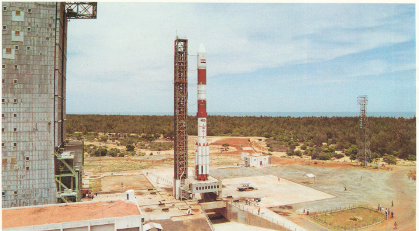
A view of the launch complex with PSLV on the launch pedestal
