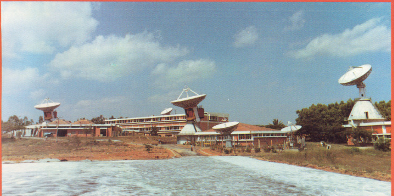
INSAT - 2 Master Control Facility at Hassan
