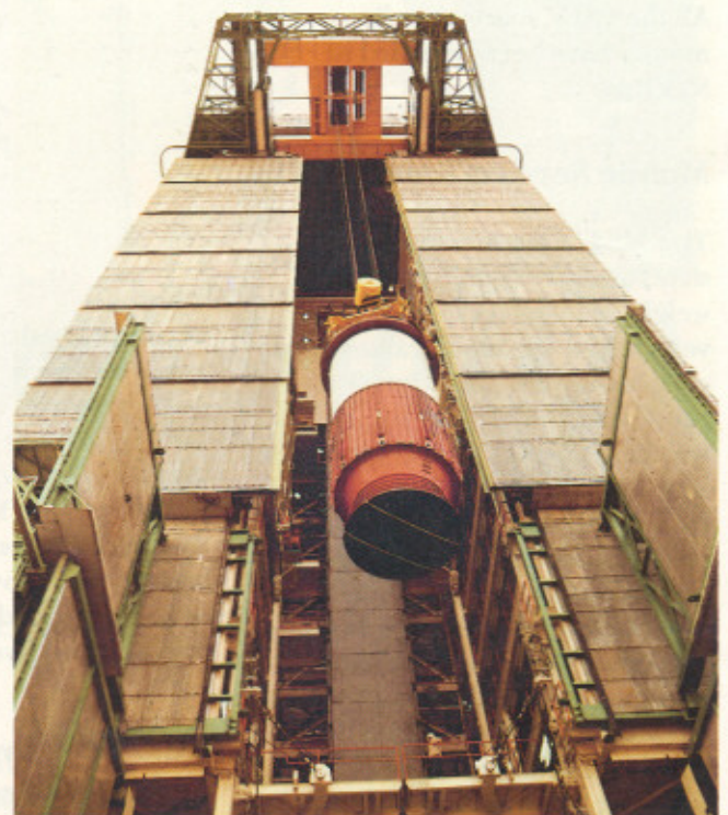
Lifting operation on nozzle end segment of the first stage motor
