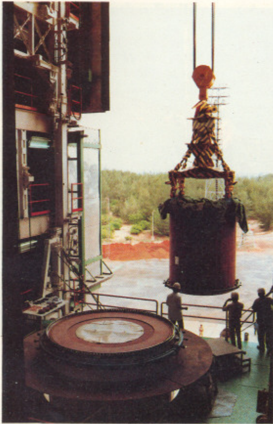
Middle end segment of the first stage being lifted for stacking on nozzle end segment
