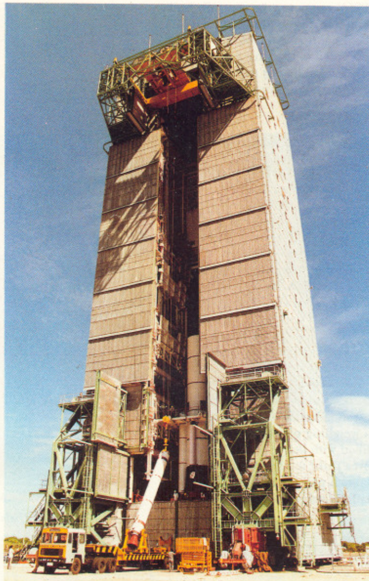
A view of the Mobile Service Tower (MST) — The loading platforms inside MST are also be seen
