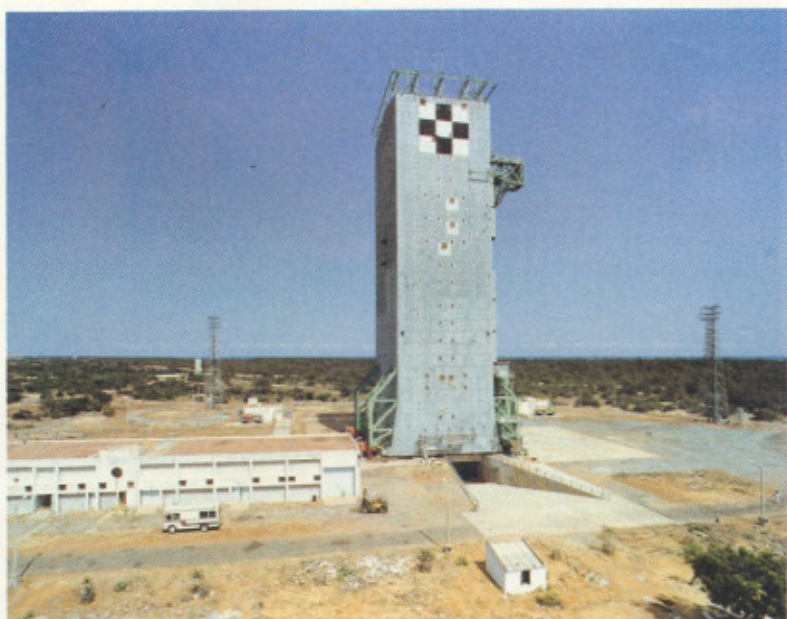
Check-out terminal room in the foreground of MST
