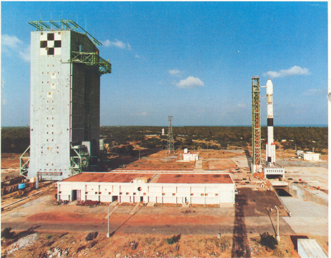
A view of the Mobile Service Tower and assembly mock-up of PSLV at SHAR Centre, Sriharikota
