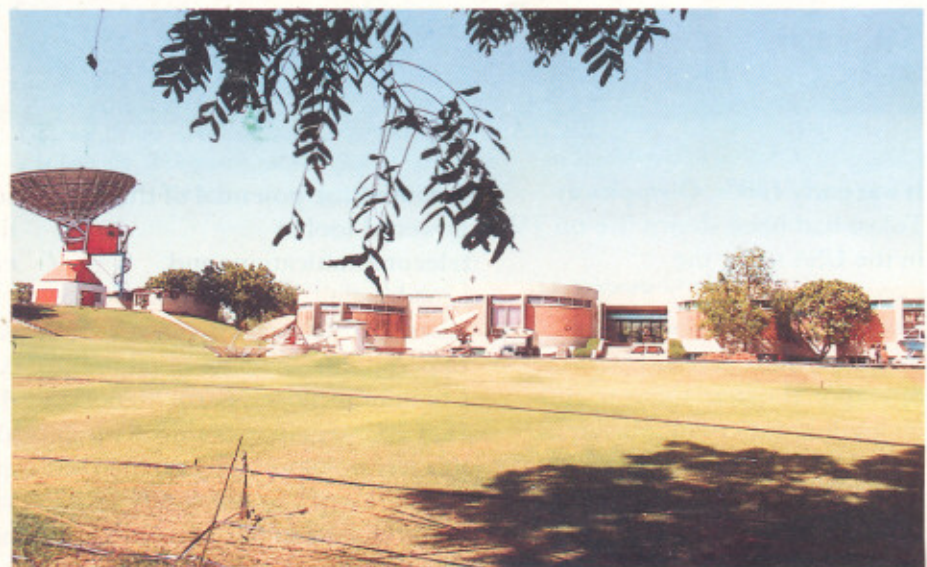
The present Ahmedabad Earth Station
