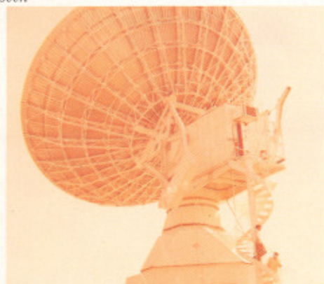
The 14 m diameter ESCES antenna
