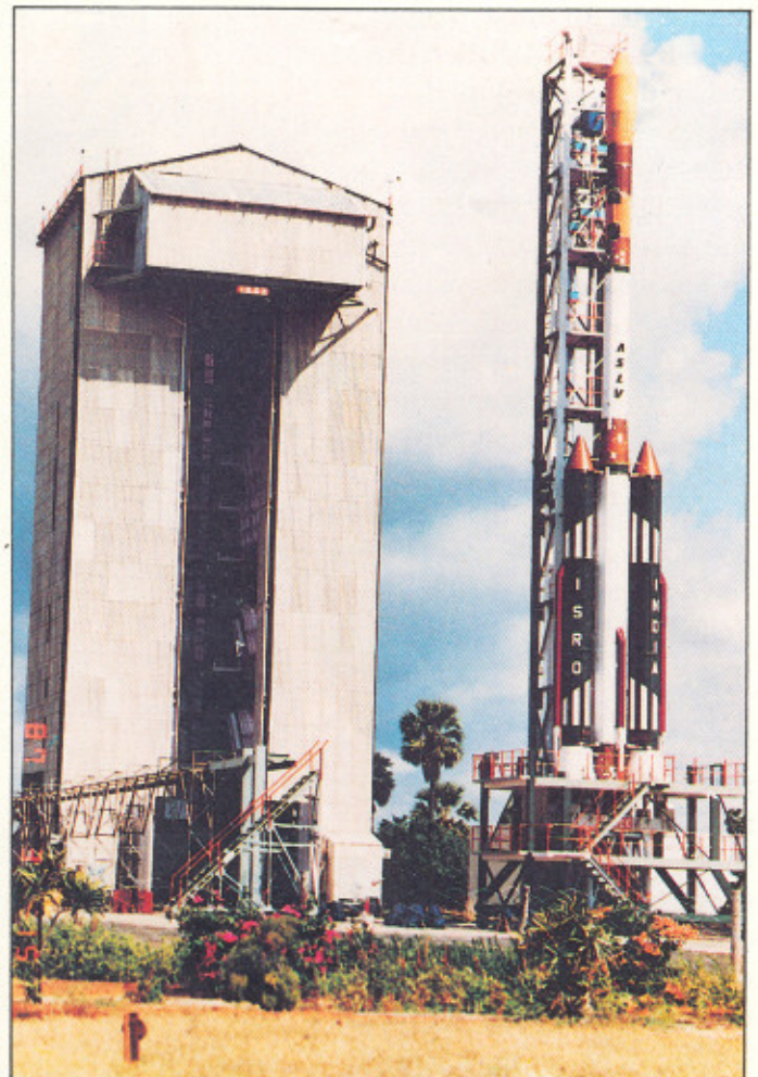
The mobile service structure being moved out
