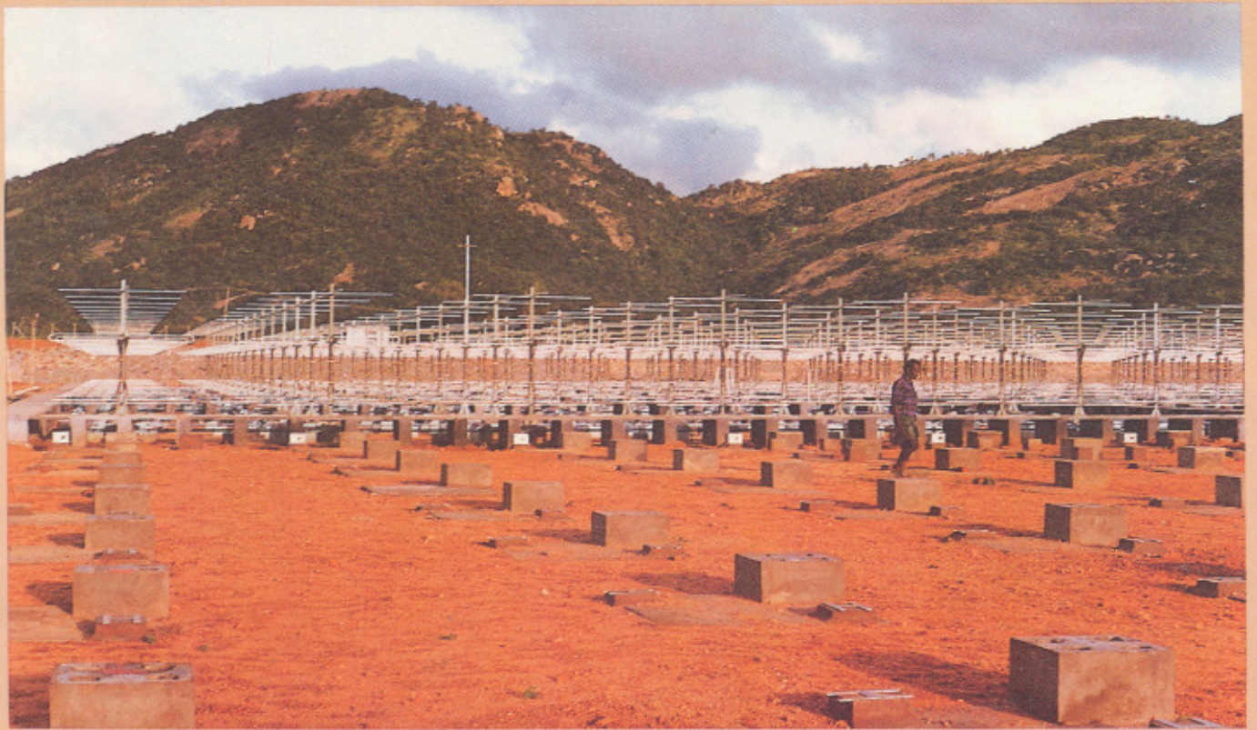
Single Element Yagi array for MST Radar
