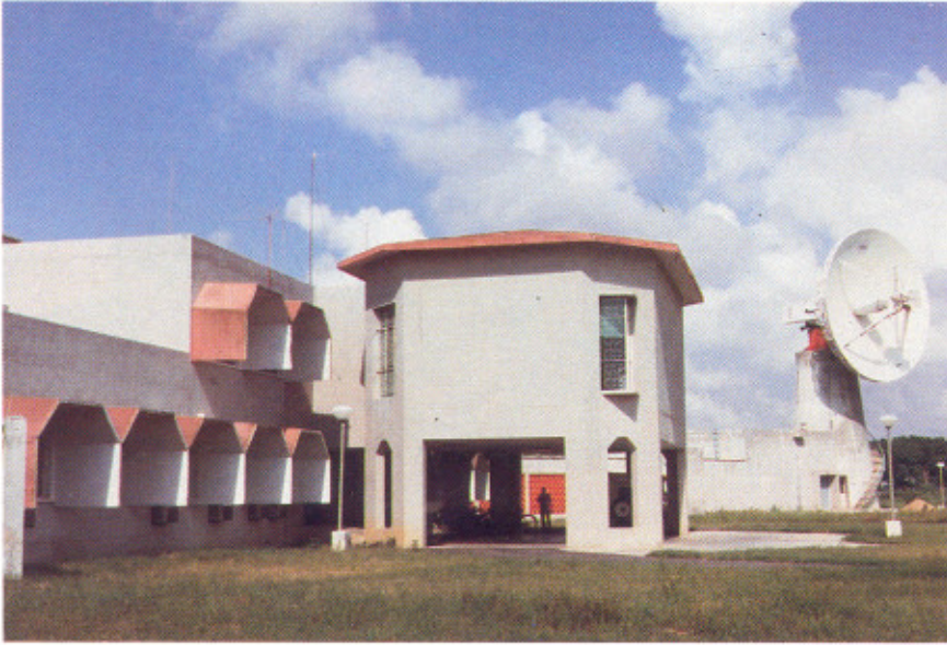
ISTRAC station at Lucknow.
