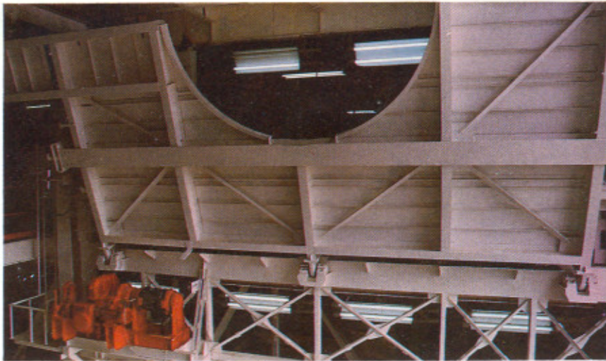
One of the foldable working platforms inside MST.
