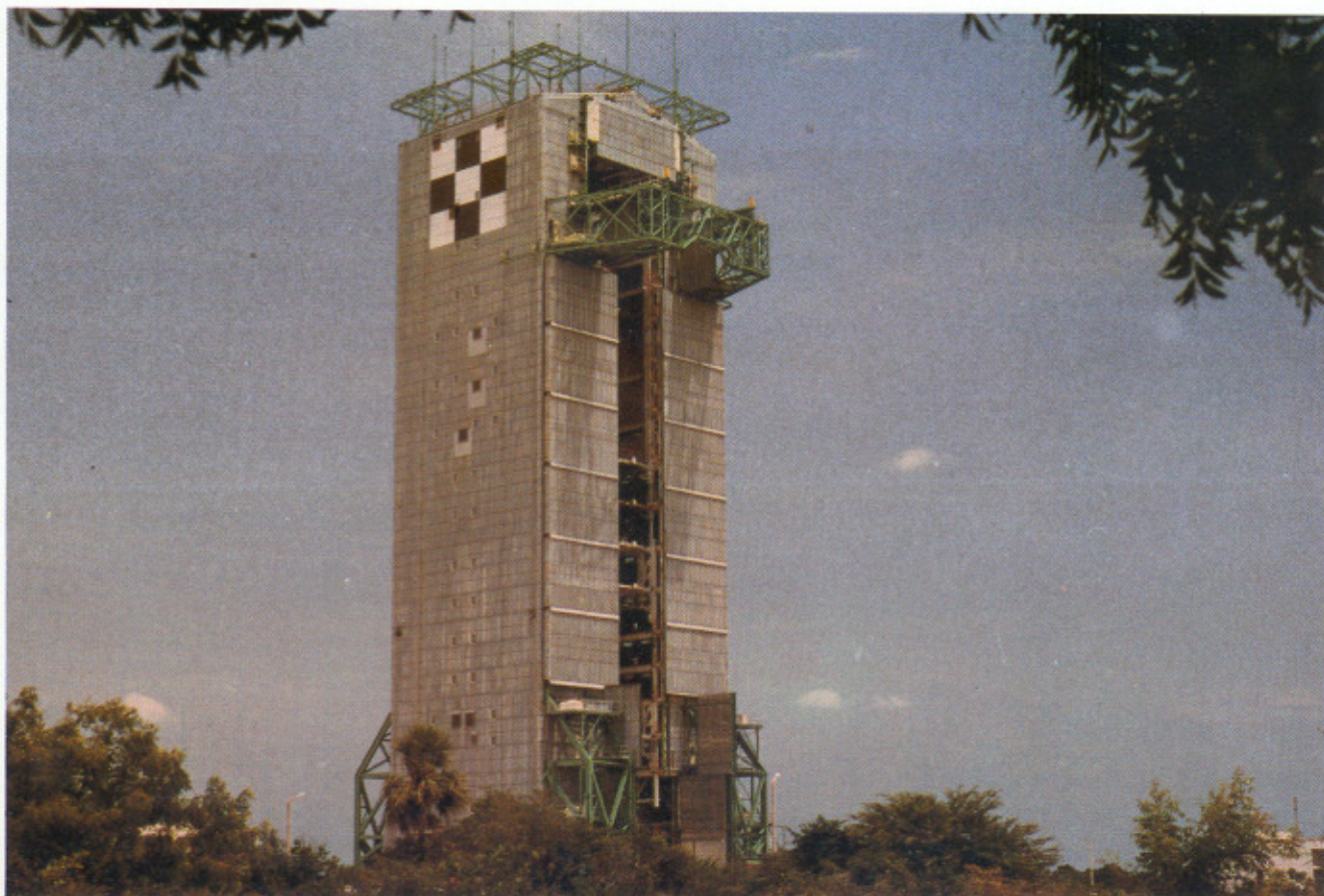
MST for PSLV - Fabrication of the tall order.
