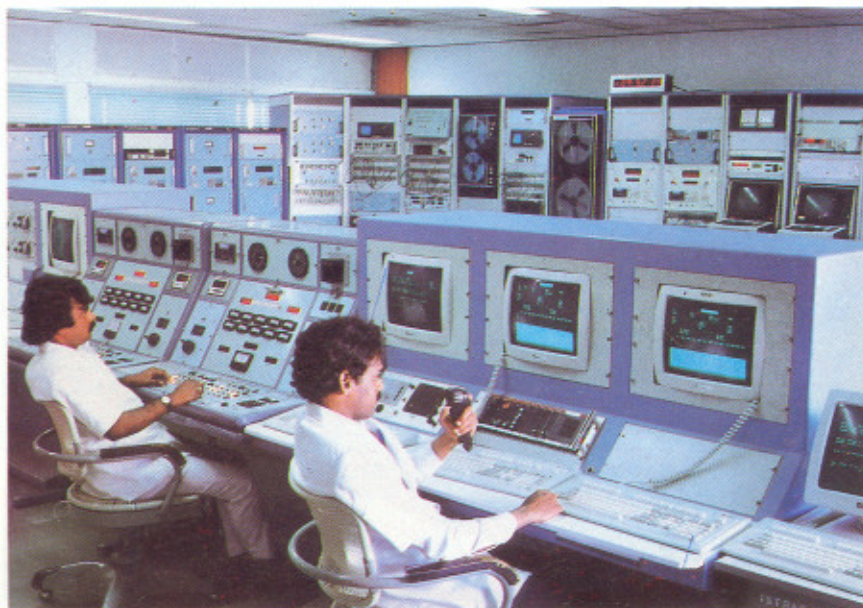
ISTRAC Ground Station at Bangalore.
