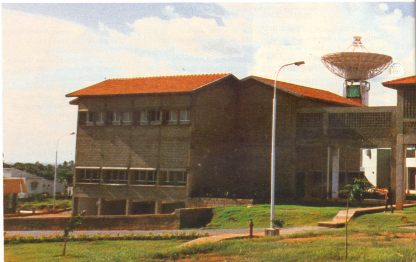
A view of ISTRAC Facilities at Bangalore.
