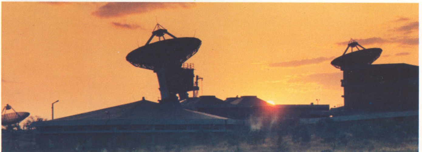
INSAT Master Control Facility at Hassan.
