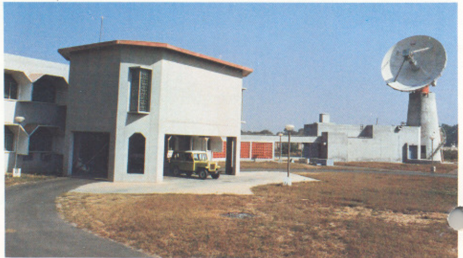
ISTRAC station at Lucknow.
