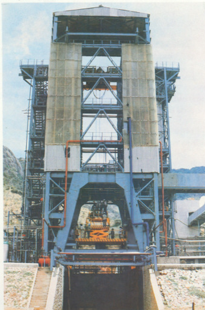
The principal test stand at LPTF, Mahendragiri
