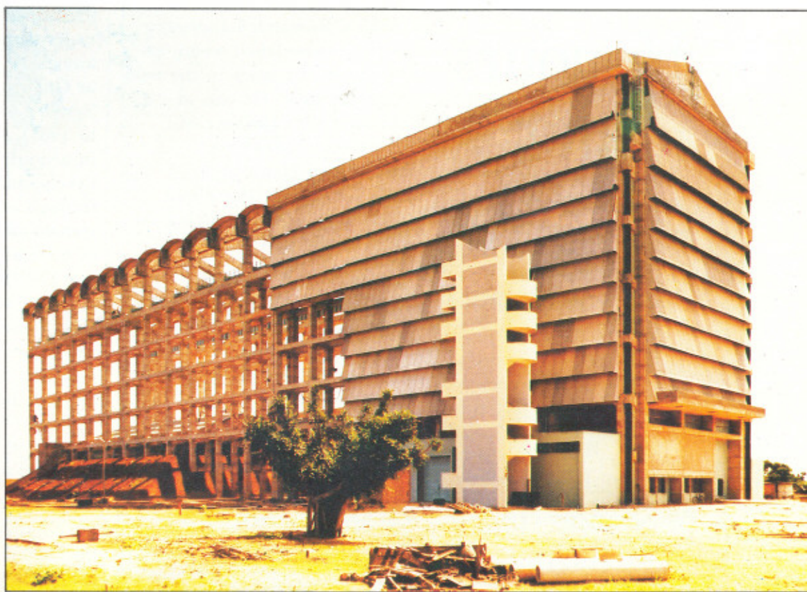
Assembly cum Static Firing Test Bay for the PSLV booster motor at SHAR Centre: This facility consists of an assembly bay, test bay and an intermediate storage area. The test area has a 12 m × 25 m RCC floor of M-20 grade concrete, designed for a dynamic horizontal thrust of 600 tonnes. The building is 126 m long, 31 m wide and 40 m high. It covers a plinth area of 1176 m 2 .
