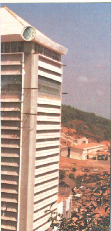
Assembly and Integration Facility at Valiamala for the dynamic testing of the full-scale models of PSLV: It consists of a stage assembly, pressure test facility, a dynamic test tower and office areas. A special cleanroom is provided for integrating some of the sub-systems. The building has a plinth area of 2621 m 2 .
