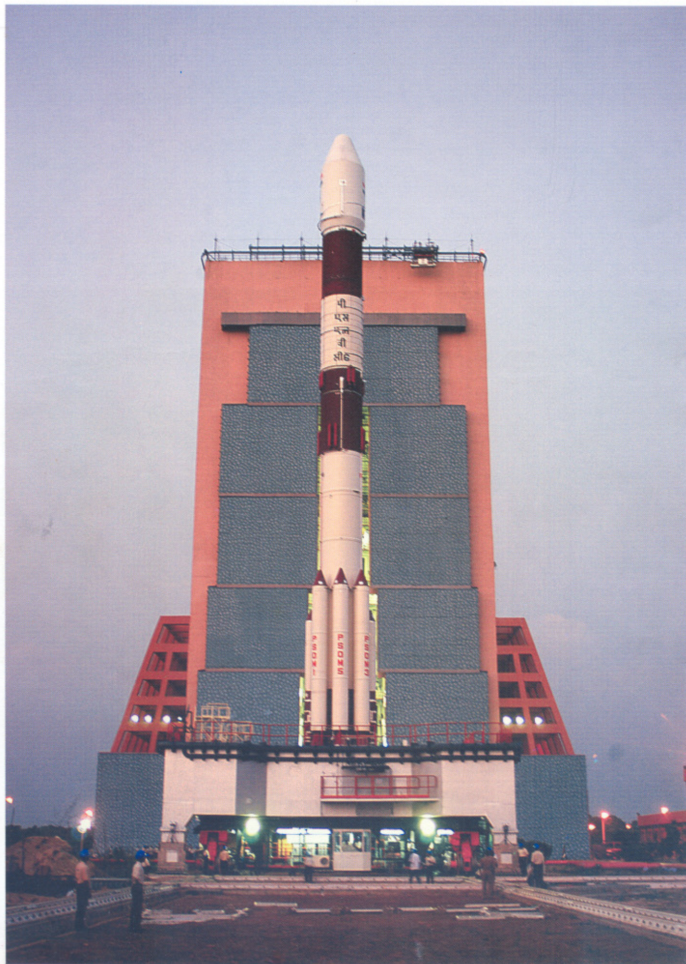
PSLV-C6 mounted on Mobile Launch Pedestal on its way to launch pad. The Vehicle Assembly Building is in the background
