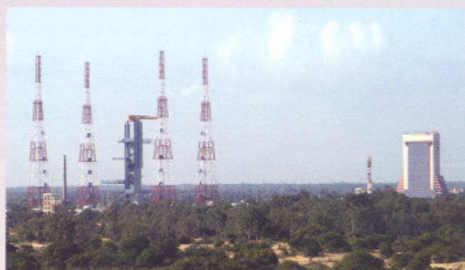
Panoramic view of Second Launch Pad showing the Umbilical Tower (left) with lightning protection towers and Vehicle Assembly Building (right)
