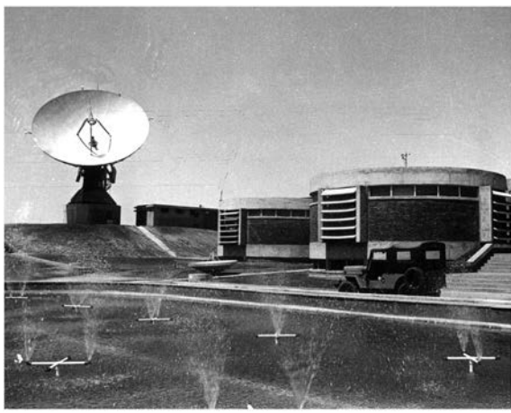
A view of Ahmedabad Earth Station beaming TV programme during SITE
